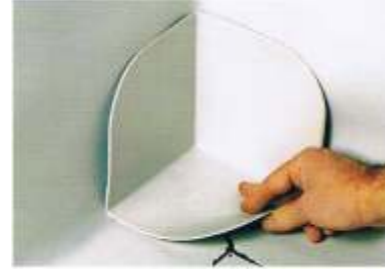
Internal corner treatment
